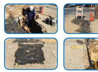
Natural gas service lines run from the main outside your home and connect to the gas meter that serves your home or business. After a new main is installed (Step 3), service lines will also need to be replaced, requiring re-excavation of the street.
