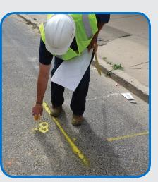
A PGW representative will mark the location of all existing PGW natural gas service lines in your neighborhood with yellow paint. The proposed excavation for new natural gas service lines will be marked in white paint. This paint is not permanent and will fade and wash away with time. Other agencies use different colors i.e. blue for water/ sewer, red for electric, orange for communications to mark the location of their utility lines.
